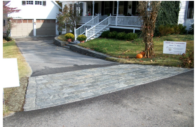
COBBLESTONE DRIVEWAY APRONS
